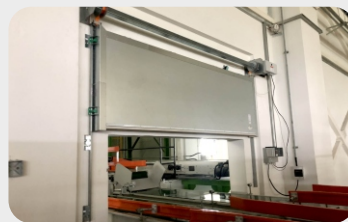
«Belarusian National Biotechnological Corporation» CJSC, Minsk region Automatic fire curtains «FireDoors», fire protection barriers of conveyor openings
