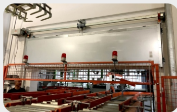
«Belarusian National Biotechnological Corporation» CJSC, Minsk region Automatic fire curtains «FireDoors», fire protection barriers of conveyor openings
